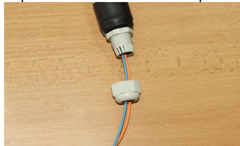
Duplex cable to be inserted into protection tube
